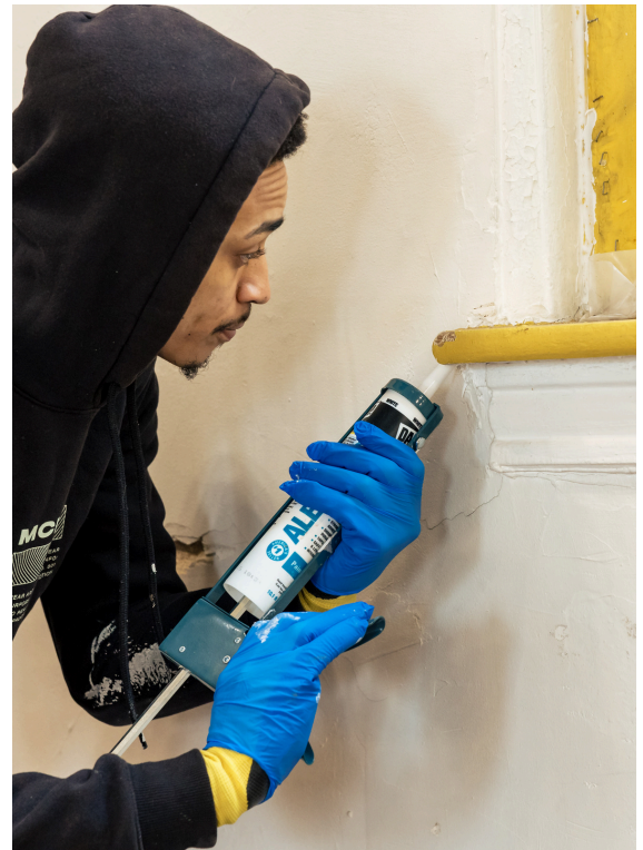
The weatherization process
